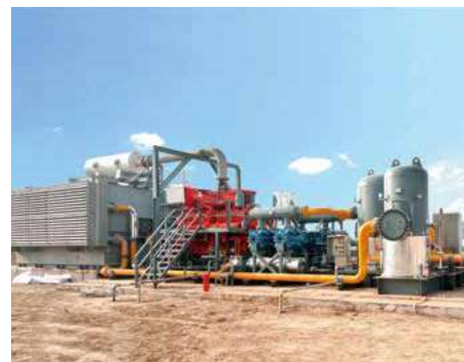
○ China ShanXi reciprocating compressor project site
