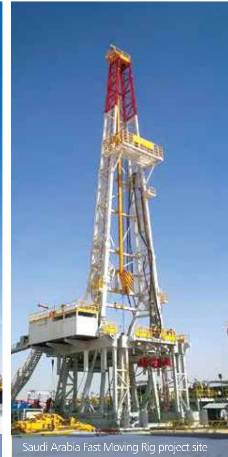
Saudi Arabia Fast Moving Rig project site
