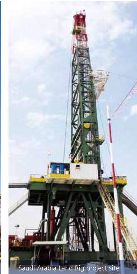
Saudi Arabia Land Rig project site
