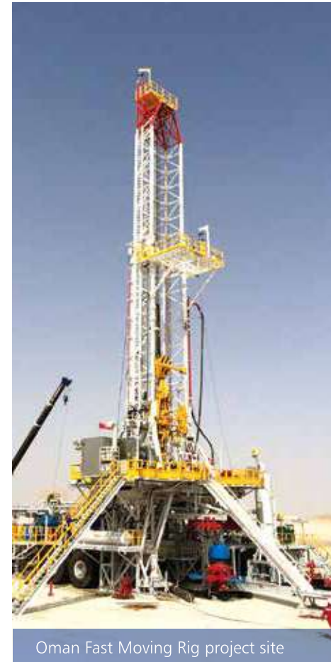
Oman Fast Moving Rig project site
