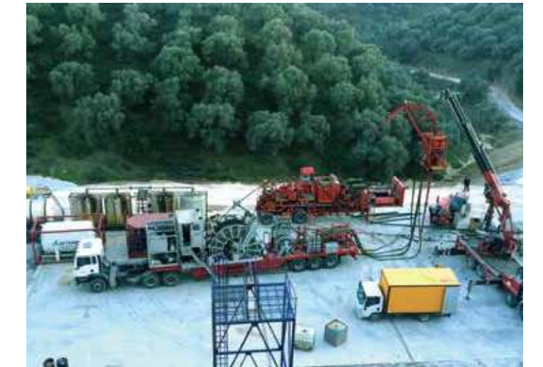
○ Turkey coiled tubing equipment working site
