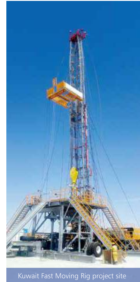
Kuwait Fast Moving Rig project site
